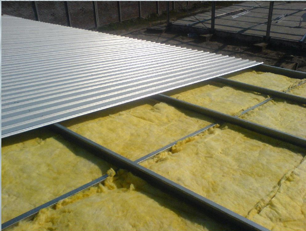
Composite layer insulation (steel color sheet+glass wool)
