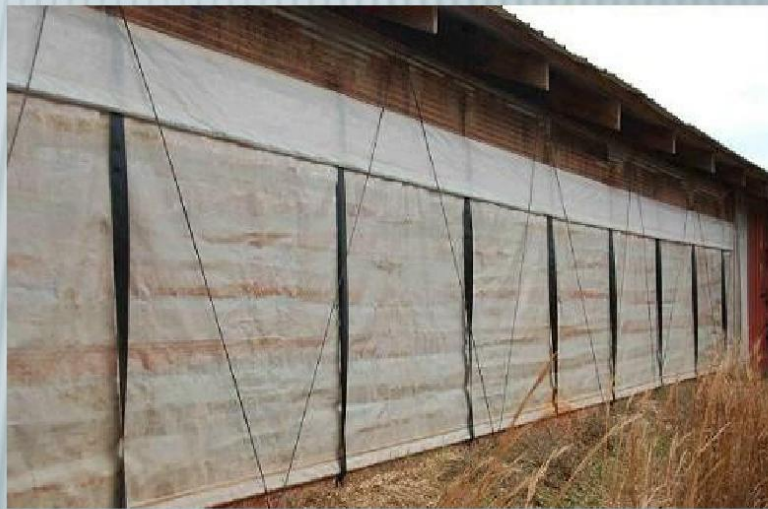
Unfixed cladding (rolled-up walls)
