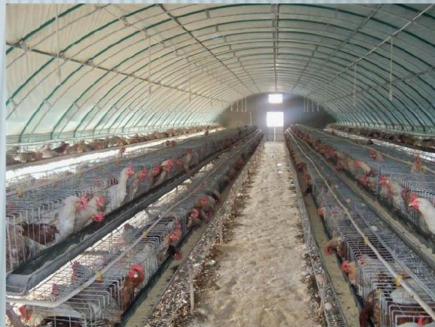
Arc roof truss poultry shed
