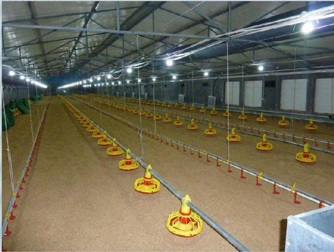
Triangle roof truss poultry shed
